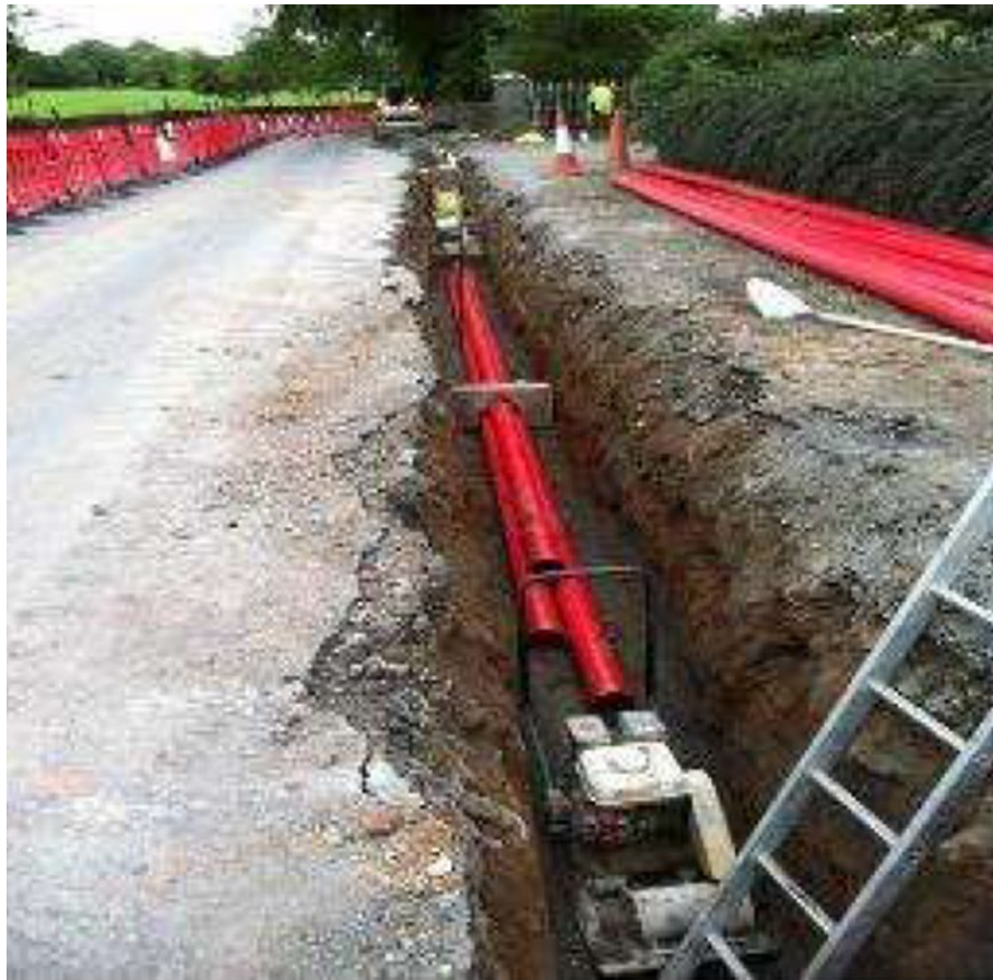
Image 2-1: Example of 110kV Underground Duct Installation
